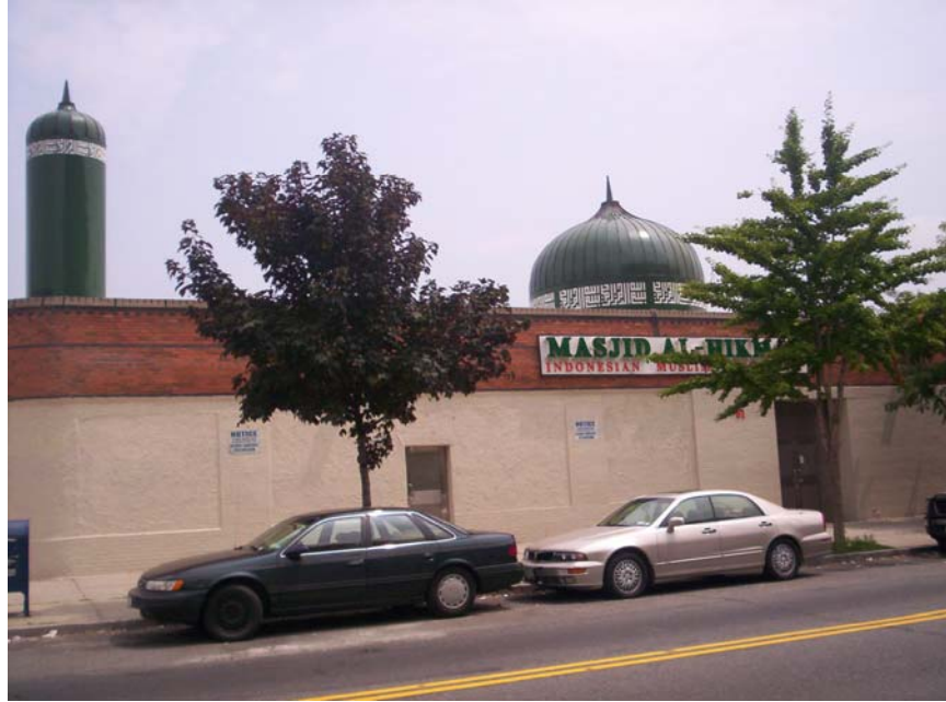
Figure 2. Front view of Masjid Al-Hikmah
